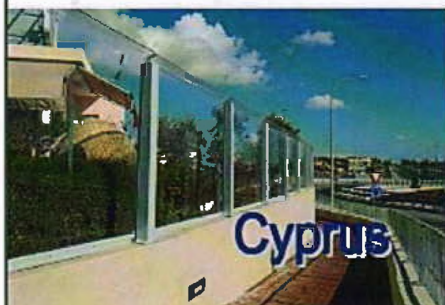
Sound reflecting noise barrier of acrylic plastic
